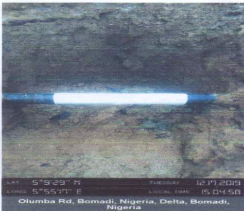
Pic 3: Repair work
